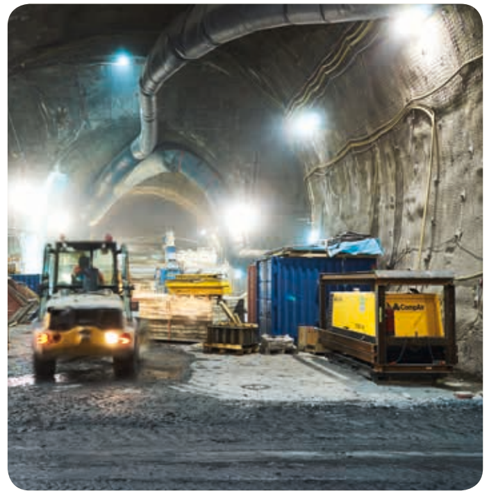
The CompAir compressor sled model follows the progress of the construction.
