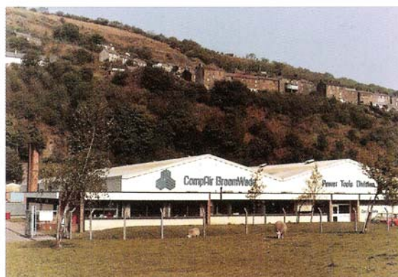
The new power tools factory in Ystalyfera, South Wales
