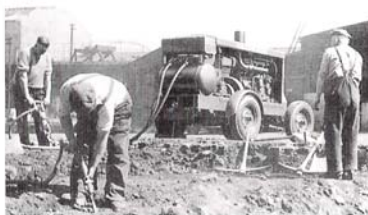
Workmen using a BroomWade portable compressor
